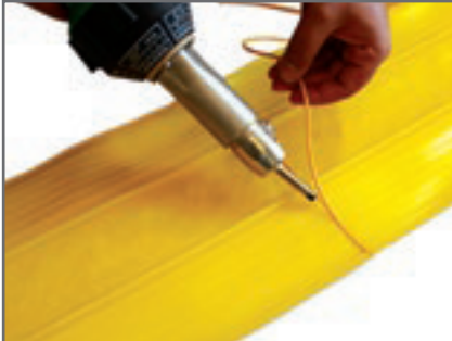
Hot air blower welding procedure
